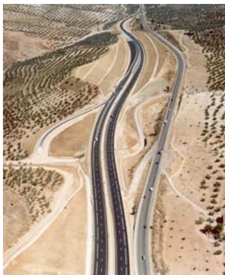
New western connection from Mancha Real to the Jaén north-west bypass.
